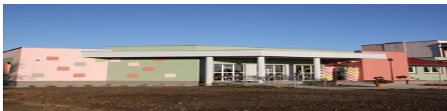
Construction of a kindergarten in Stare Oborzyska
