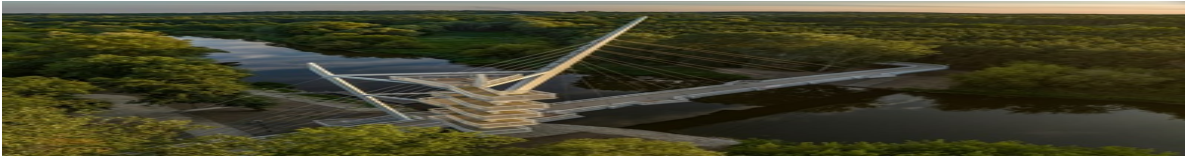
Expansion of the pedestrian and bicycle path system in Owińska together with the construction of a pedestrian and bicycle footbridge over the Warta River
